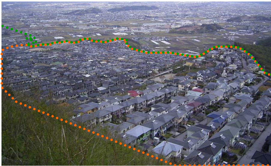
View of service area from an AP
