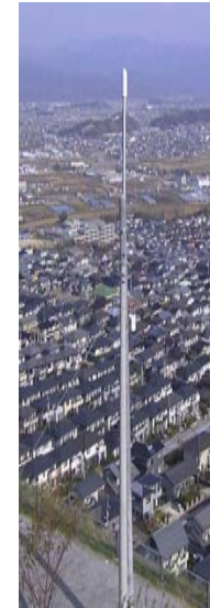
AP on an electrical pole
